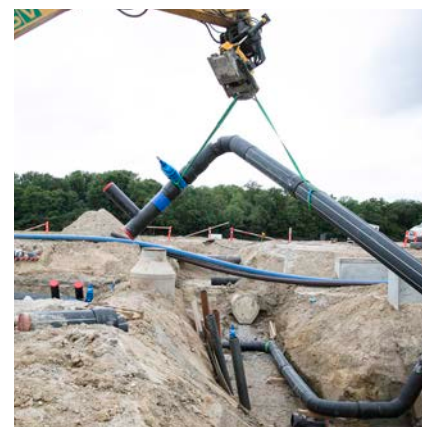
Easy handling and installation PE pipes are easy to handle and transport, and welding can be done above ground.
