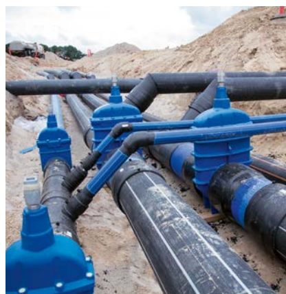
Flexible material PE pipes are flexible and follow the terrain, so there is no need to level the soil in the trench.
