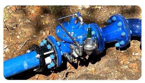
The pressure variance for this section of the network was 5 bar to 2 bar, with a flow range of 2-17 litres per second. Following the valve replacement, the AVK UK PRV is maintaining this benchmark and has even improved readings from the critical point logger, bringing pressure variance down from 6 meters to 3 meters over the previous two months, which will aid in reducing leakage rates.
