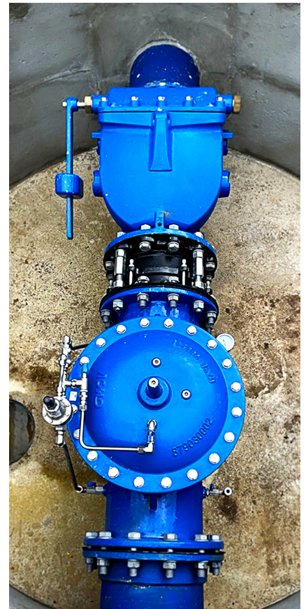
Pictured is the pumping station, and inset, the chamber housing a AVK UK DN300 Series 41 Swing Check Valve, and a DN300 Series 879 Pressure Sustaining Valve (PSV).
